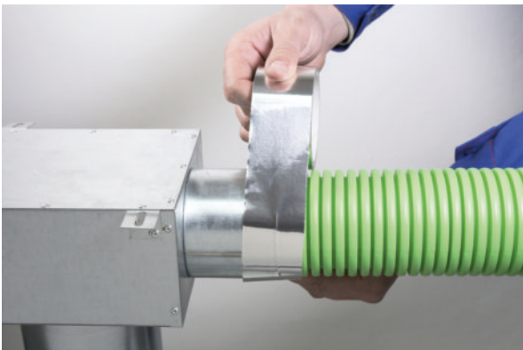
7) Secure the connection using air-tight self-adhesive tape.
