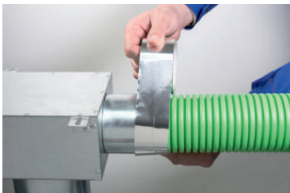
7) Secure the connection using air-tight self-adhesive tape.
